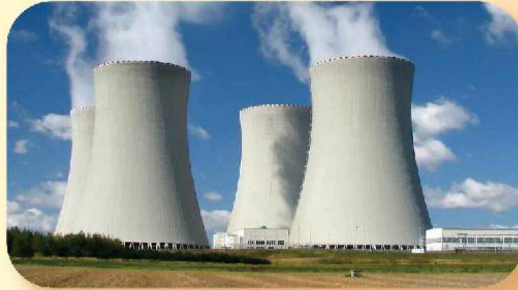
NUCLEAR POWER PLANT
